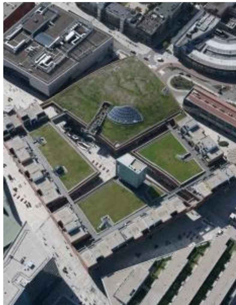
Centre Commercial a Bruxelles
